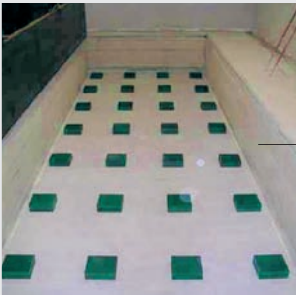
Verlorene Schalung, "Lost form working technology"
